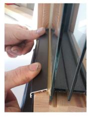
Push the front edge down so that the Aluminium capping keys into the clear plastic clips
