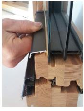
Now push the capping edge facing the glass onto the clips
