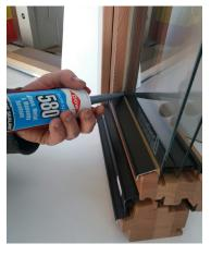
After the capping profile is fixed, use black neutral cure silicone to seal inbetween capping and glass
