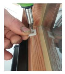
Screw the clips to the sash profile with 3x20mm countersunk stainless steel screws
