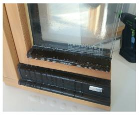
Apply plenty of separating agent on the Aluminium and timber surface (or dishwasher liquid mixed with water). This avoids that the silicone sticks to those surfaces
