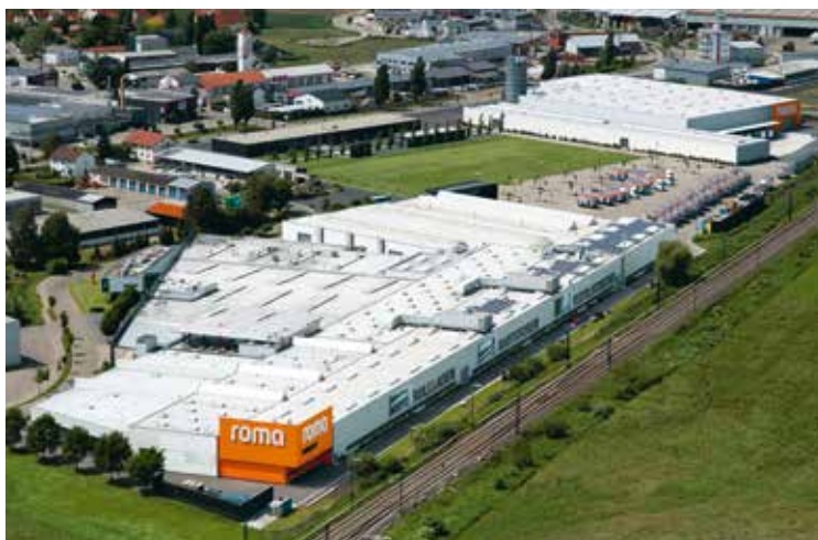
The ROMA headquarters and factory in Burgau
